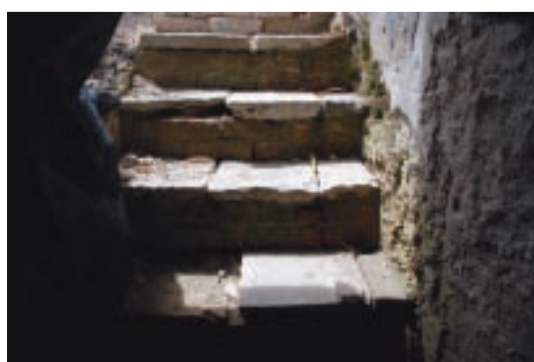
The Mikvah, the water is constantly pumped out
